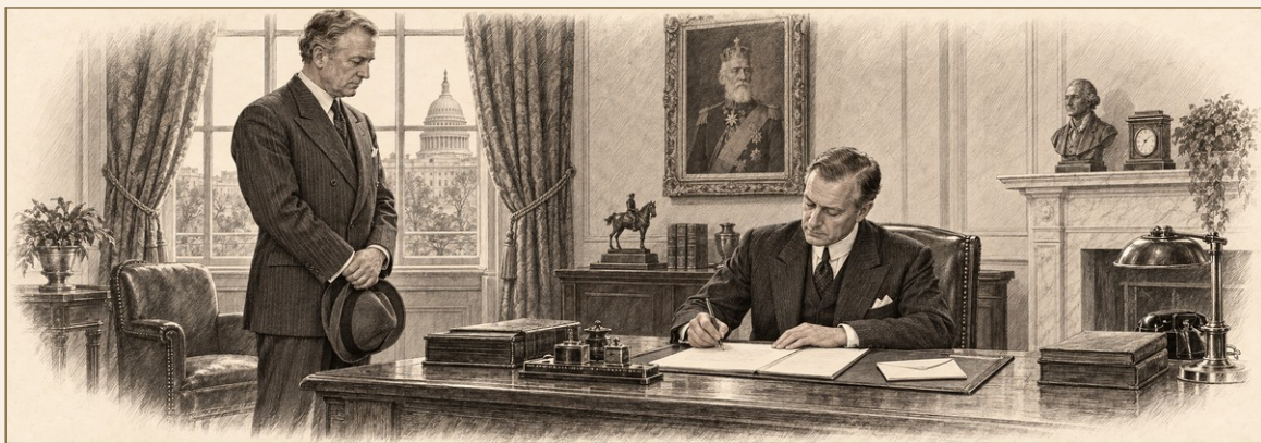
Figure 3.1: Washington, 9 April 1941. The Department's reconstruction. The minister signs. The instruction not to has not arrived, and would not have been followed.
